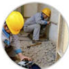
Building grounding measurement
