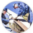
Grounding grid measurement
